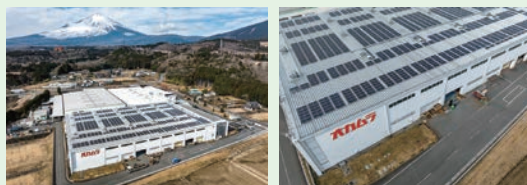
Solar panels at the Gotemba Plant
