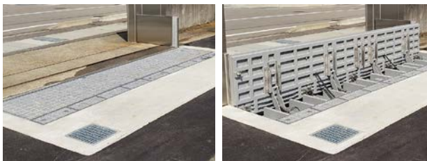
The electrically operated raisable flood barrier SuiZin (left: under normal conditions, right: with the flood barrier raised)
